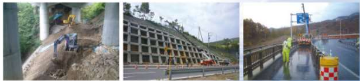
清風橋下部法面補修
